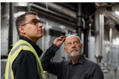
HVAC | Air handling units Fan coil units
